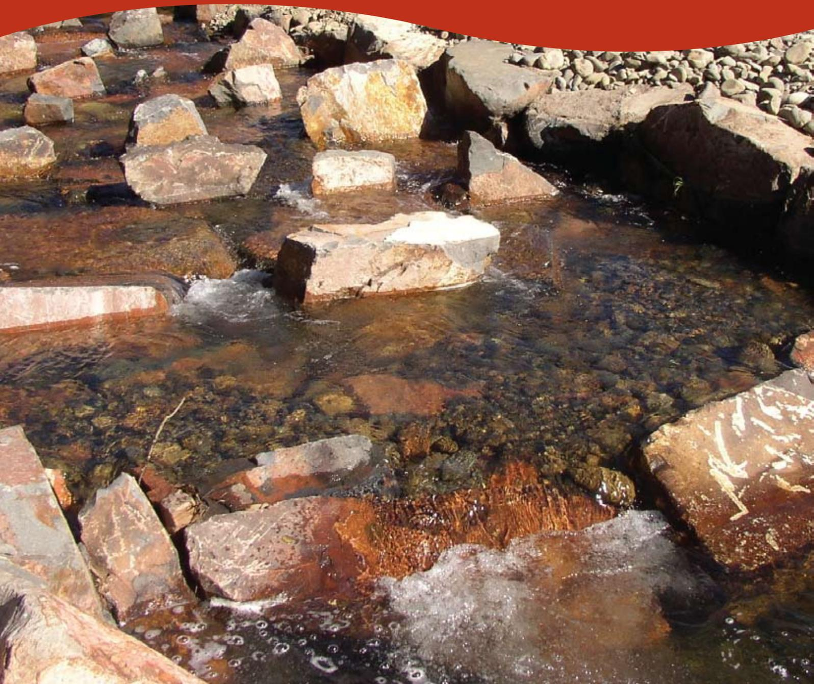
*Modern fishways are custom designed to incorporate resting pools into areas where water has a high velocity, allowing the fish to use a burst of speed to progress upstream. Photo: Industry and Investment NSW.*
